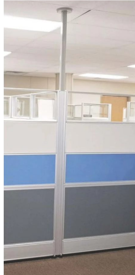
Ceiling power pole when installed
